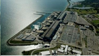
Pickering Nuclear Power Station
