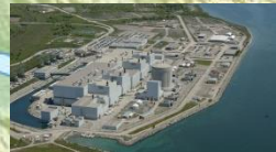
Darlington Nuclear Power Station
