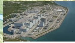
Darlington Nuclear Power Station
