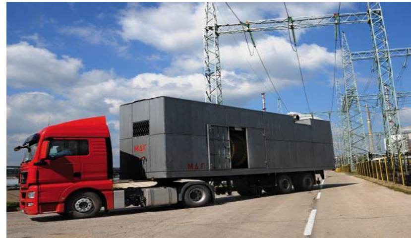
Mobile Diesel Generator (MDG) P=1.1\text{MW} , 6kV
