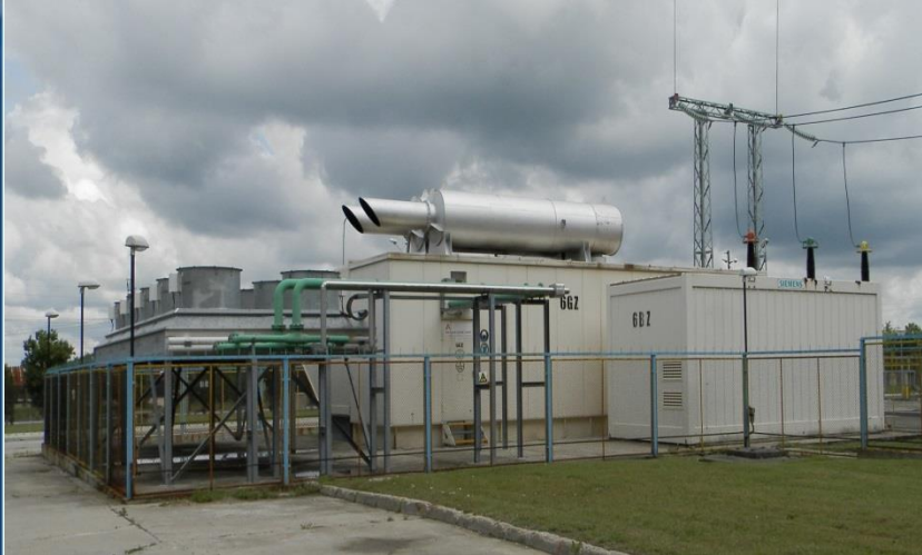
Auxiliary Diesel Generator (DG), module type, stationary. P = 5.4\text{MW} , 6kV
