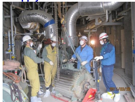
Replacement of a motor
