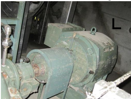
Water damage on motors induced by tsunami TOKYO ELECTRIC POWER COMPANY
