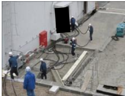
Laying temporary cables
