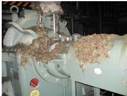
Water damage on pumps induced by tsunami
