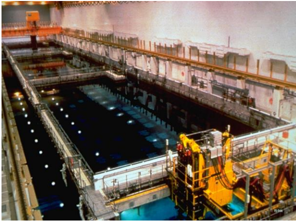
Fuel Handling Plant
