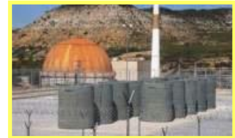
INDEPENDENT SPENT FUEL STORAGE INSTALLATION (ISFSI)
