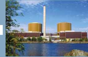
Loviisa power plant
