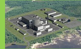
In NPP site:
