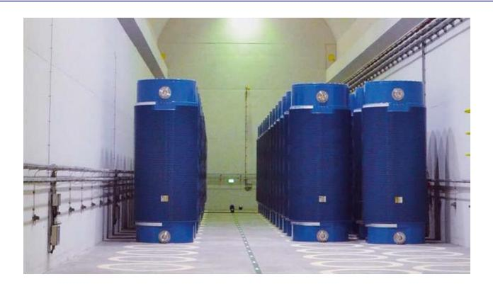
In Germany spent fuel is stored in dual purpose casks (DPCs). The transport package design approval is maintained over the whole storage period.
