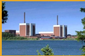
Olkiluoto power plant
