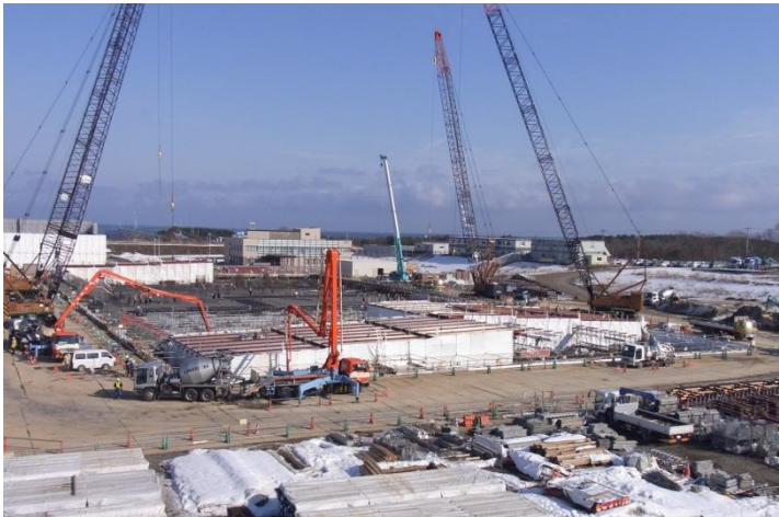
Feb. 2011 (Construction rate: about 45%)
