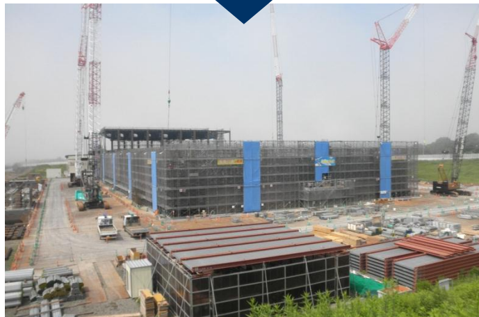
July 2012 (Construction rate: about 65%)
