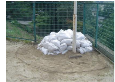
Sandbag the burlap sacks for radiation shielding
