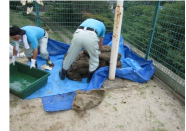
Put residue in burlap sacks. The sacks are folded and stacked on a water sealing sheet
