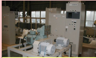
(7) Electric Motor Test Facility
