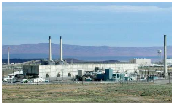
U-Canyon at Hanford (ISD Project)
