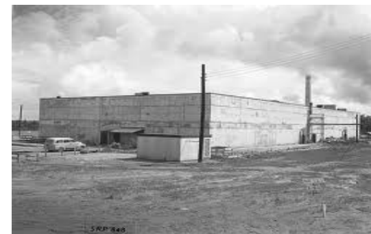
235-F Building at Savannah River Site (Deactivation Project)
