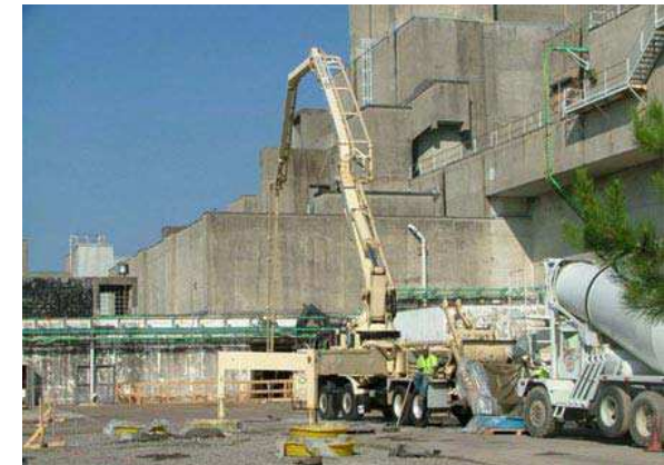
Specially engineered grout fill being pumped into a Savannah River P Reactor building
