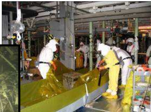
Holding basin for spent nuclear fuel
