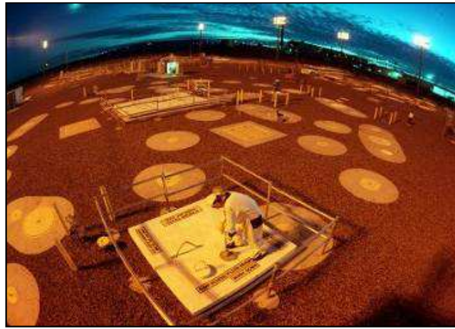
. . . Safely storing it in 200+ underground tanks . . . and
