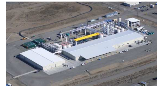
Pump and Treat Facility
