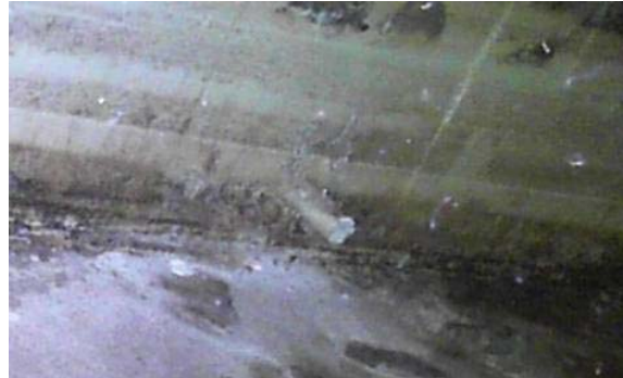
Edge of sand cushion drain pipe
