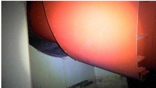
Edge of vent pipe sleeve
