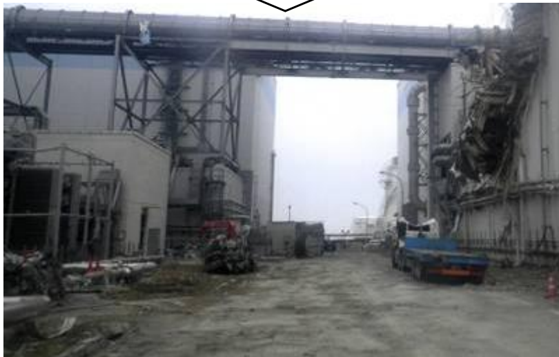
Between Unit 2 and 3
