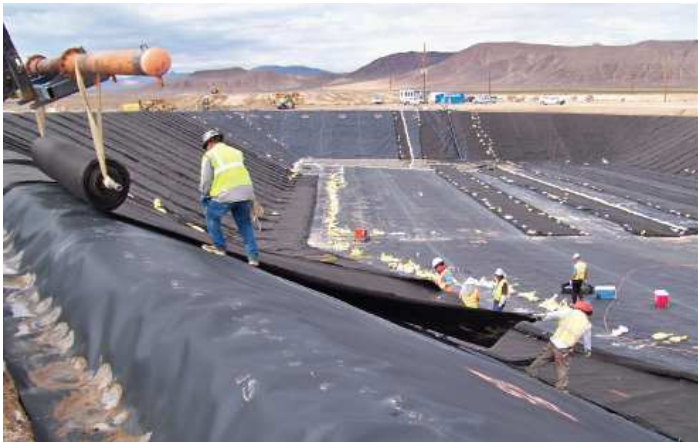
Installation of liner at Nevada Site
