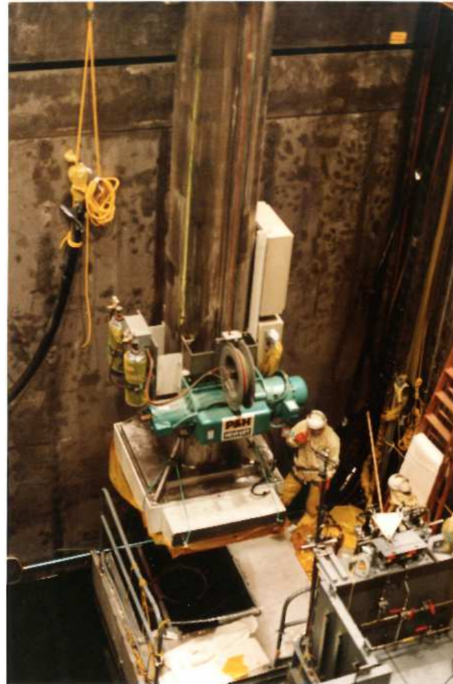
Transfer Cask Operations
