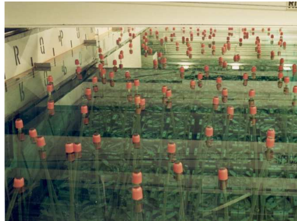
1990 to 2000 Wet Storage in Spent Fuel Storage Pool
