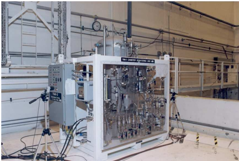
Canister Dewatering Machine in the Pool Area
