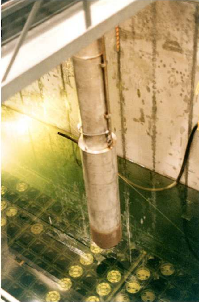
Canister Staging in Spent Fuel Pool
