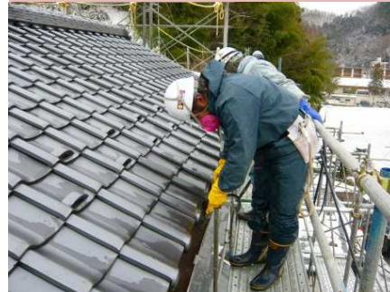
堆積物の除去 Removal of sediment
