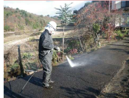
高圧水洗浄 Washing with high pressure water
