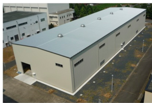
Fig.10 PF coil manufacturing building with a 80 m long which was completed at the JAEA Naka site in March 2009
