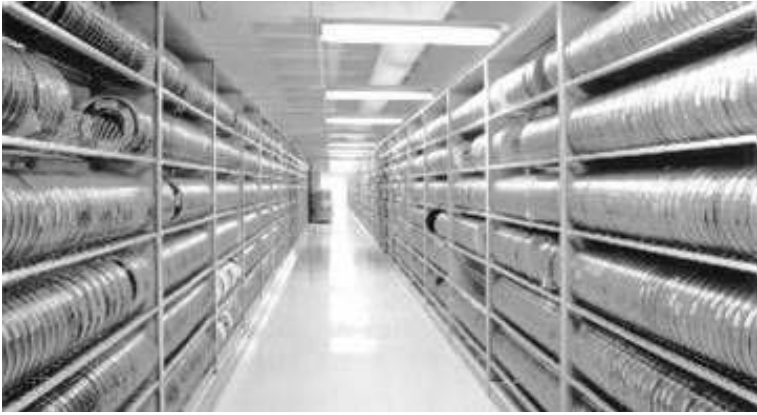
FIG. 4. A typical storage facility for computer tapes, depicting the required level of environmental controls.
