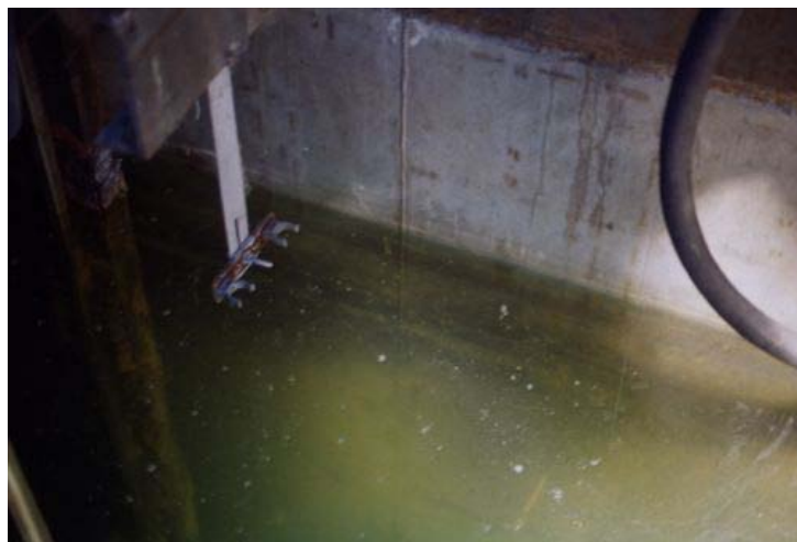
FIG. 45. Water surface of the spent fuel storage pool.
