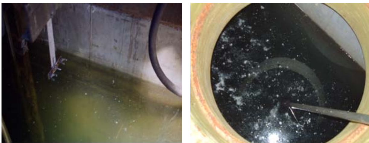
FIG. 11. Spent fuel storage facilities with solids floating on water surface.
