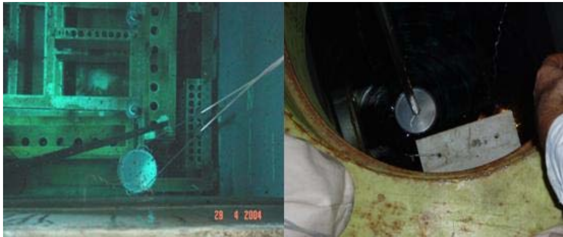
FIG. 15. Photographs showing the position of the collectors in: the reactor pool in Thailand (left) and the spent fuel basin in Romania (right).
