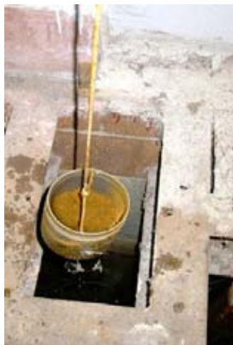
FIG. 17. A bucket of sludge being removed from the bottom of a spent fuel storage basin.
