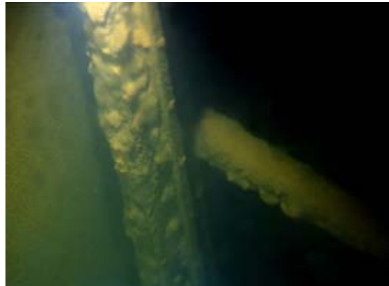
FIG. 44. Corroded steel structure inside of spent fuel storage pool.
