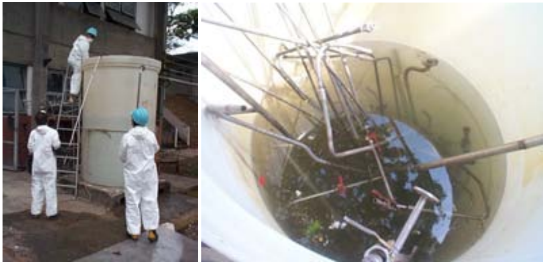
Fig.22. Polypropylene tank adapted for decontamination of large steel pieces.
