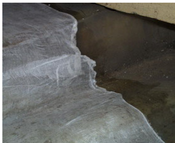
Fig. 14. Example of application of reinforced polymeric protective film on the stair.
