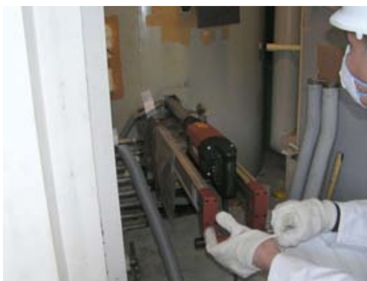
Fig. 8 Drilling a core around the drainpipe
