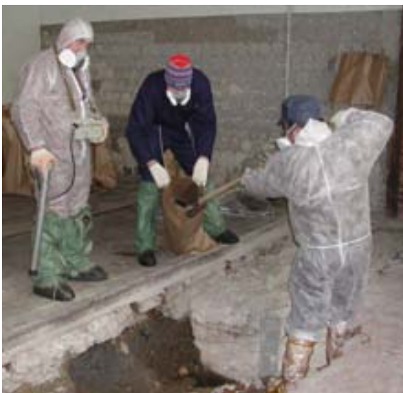
Fig. 17. Packaging of radioactive wastes on-site.
