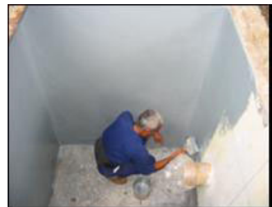
Fig. 23. Repairing the walls and floor of the retention tank.
