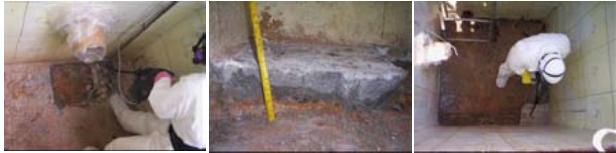
Fig. 16. Dismantling operations in the bottom of the retention tank.
