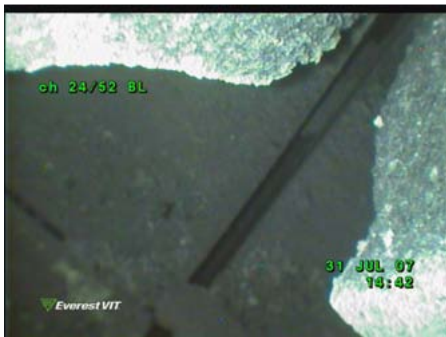
Fig. 11. Oxidation damage in the graphite structure at channel 24/52 BL.
