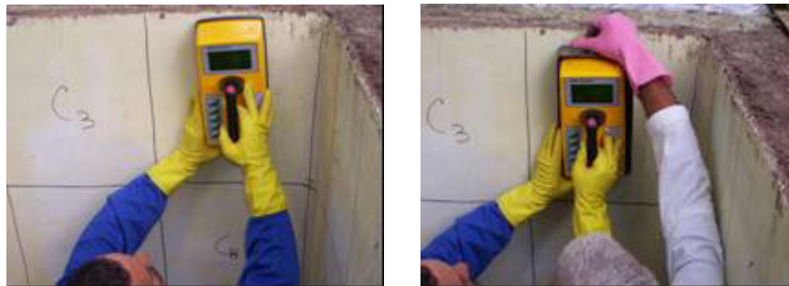
Fig. 15. Surface contamination monitoring inside the retention tank.
