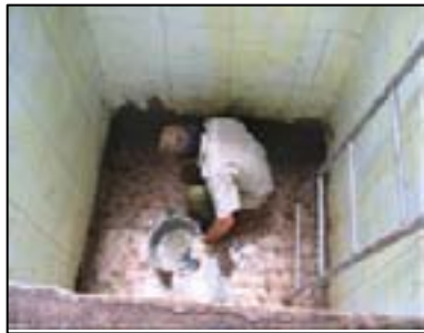
Fig. 23. Repairing the walls and floor of the retention tank.
