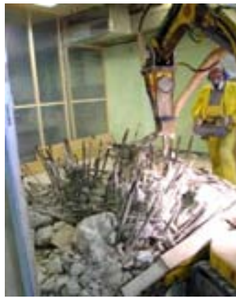
Fig. 11. Reduction of blocks dissected at activated zone.
