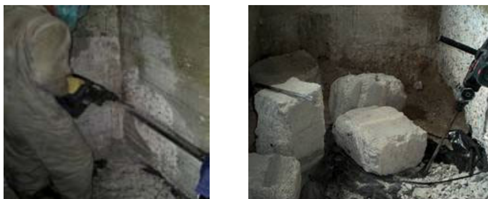
Fig. 2. Dismantling operations inside the rooms.
