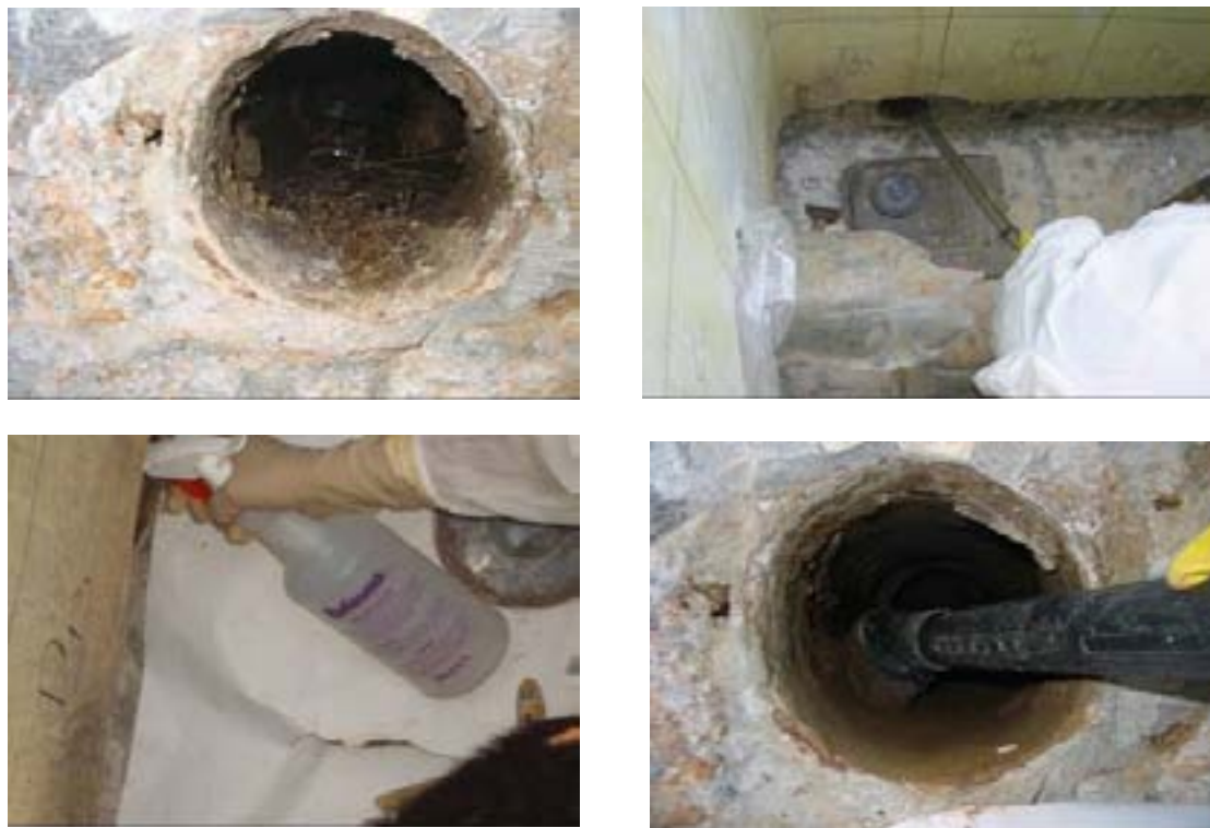
Fig. 19. Decontaminating the pipes.
