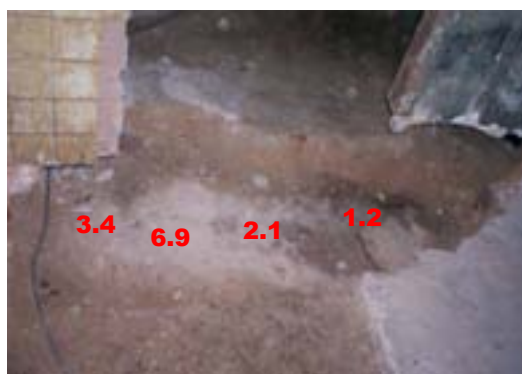
Fig. 3. Dose rate levels ( \mu\text{Sv/h} ) remained in a contaminated area of room 7.
