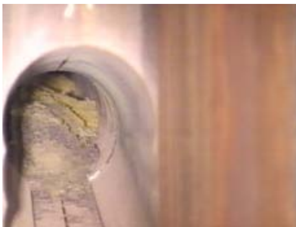
Fig. 4. Fire damaged fuel element displaced from its graphite boat.
