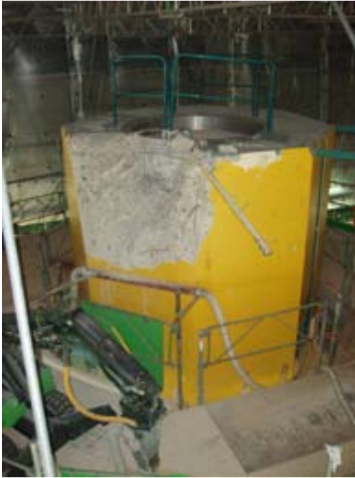
Fig. 21 Start of demolition from platform.
