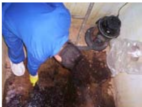
Fig. 13. Collection and storage of radioactive effluents from the retention tank.
