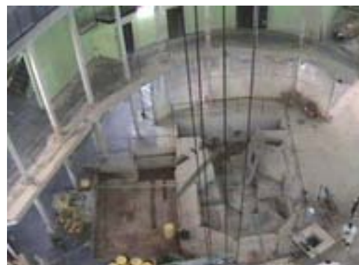
Fig. 17. Removing of primary tubing embedded within foundations of the biological shield.
