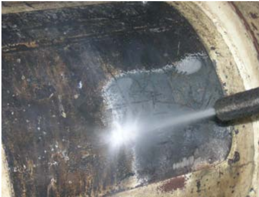
Fig. 4. Decontamination by dry ice blasting.
