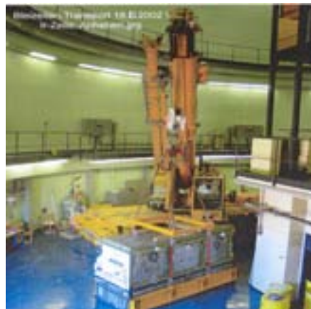
Fig. 2. Clearing the reactor building, transfer of a 21-ton lead cell.
