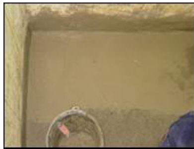
Fig. 23. Repairing the walls and floor of the retention tank.
