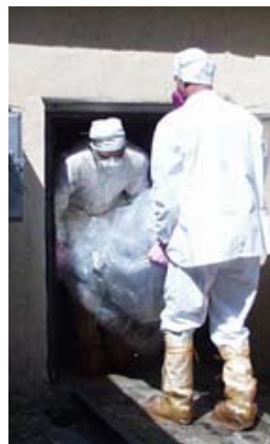
Fig. 18. Transportation of RAW to on-site temporary storage.
