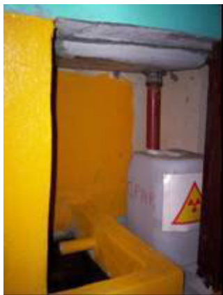
Fig. 10. Temporary system for collection of possibly contaminated effluents at the WPF.
