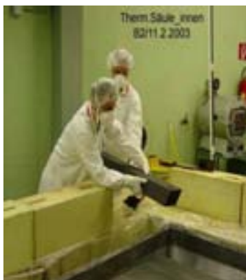
Fig. 3. Inner thermal column, recovering of the graphite.
