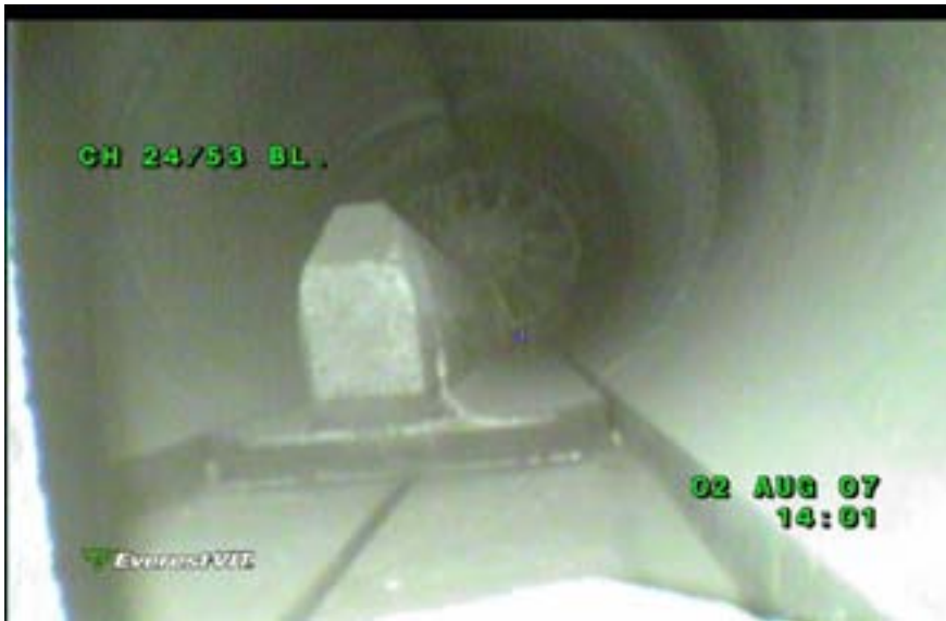
Fig. 9a. Fuel channel 24/53 BL internals showing fuel element displaced from graphite boat.
