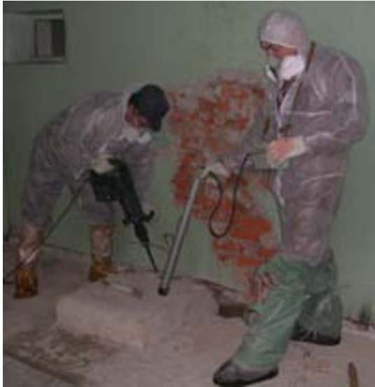
Fig. 15. Decontamination of concrete with handy tools.
