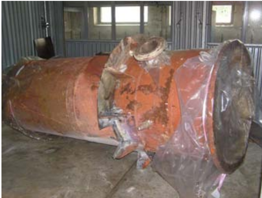
Fig. 11. Heater before dismantling.
