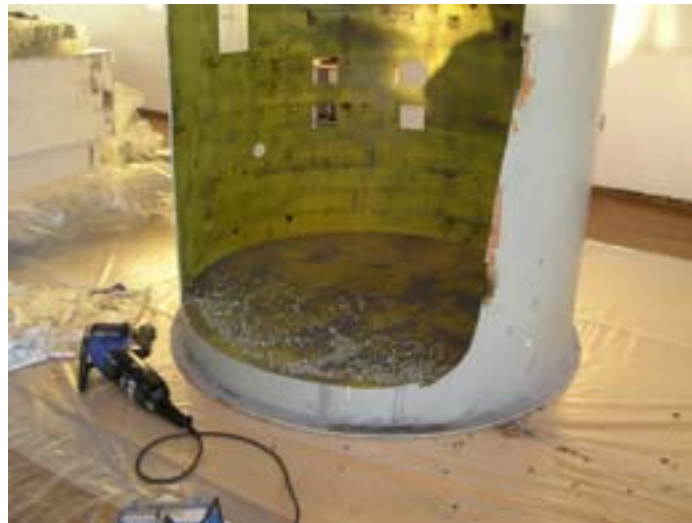
Fig. 13 The nibbler and the half-cut reflector tank.
