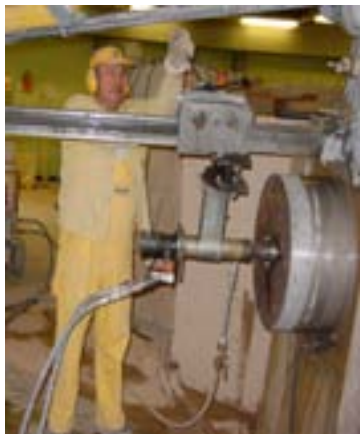
Fig. 10. Attempted core-drilling at the beam tubes.
