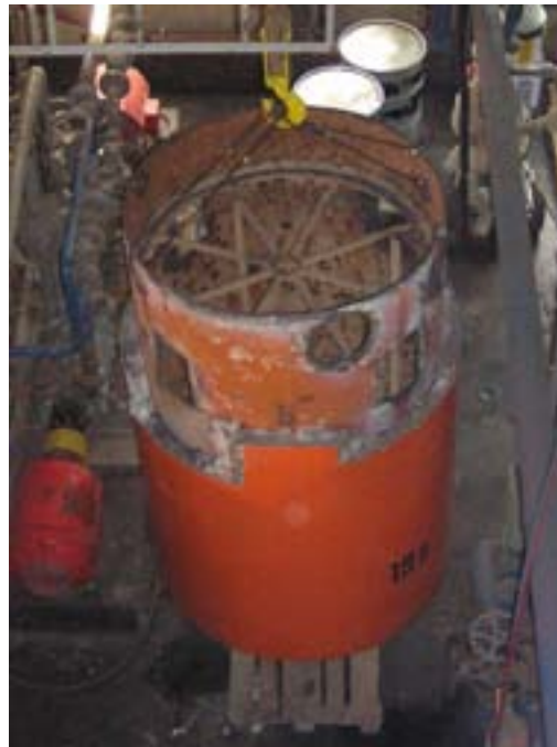
Fig. 8. Separator removal.
