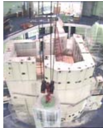
Fig. 6. Removing of blocks 1 st layer.
