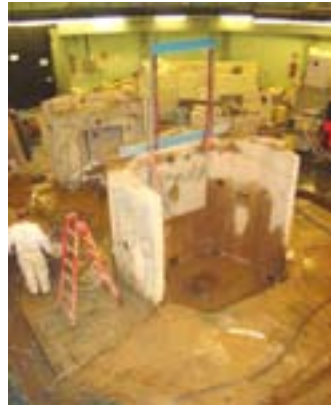
Fig. 15. Biological shield; Activated zone remaining.
