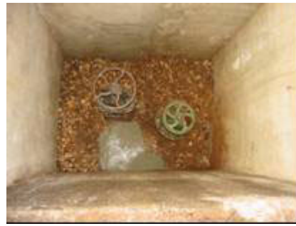
Fig. 22. Closing a ramification of the outlet pipe.
