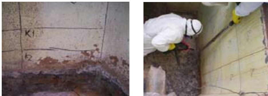
Fig. 17. Dismantling operations in the walls.
