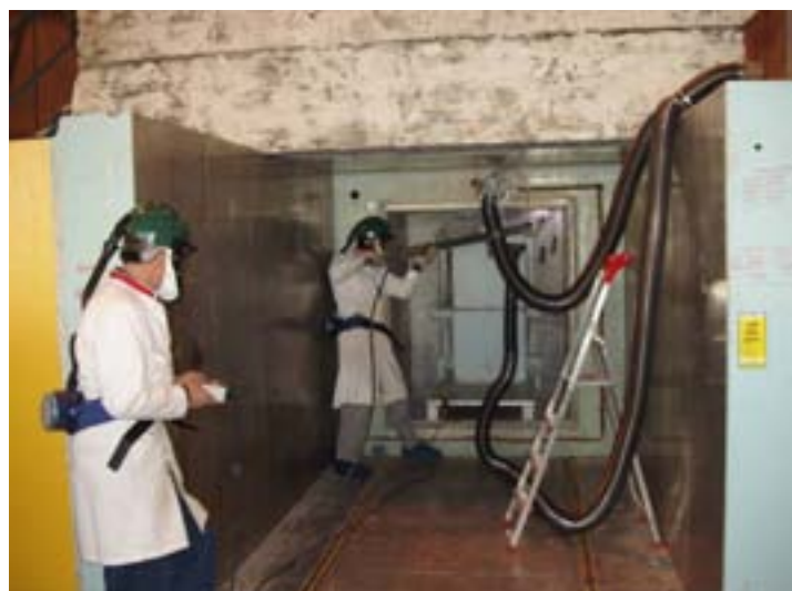
Fig. 18 Plasma cutting of the lead nose.
