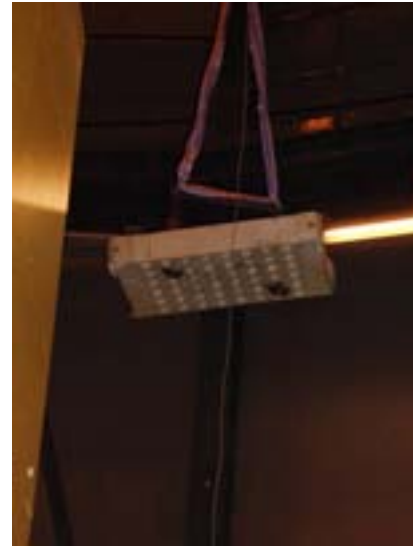
Fig. 20 Grid plate hanging in crane.
