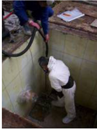
Fig. 20. Use of vacuum cleaner to avoid the dispersion of contaminated powder.
