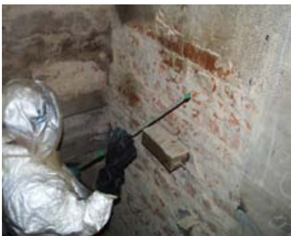
Fig. 13. Treatment of contaminated concrete with dust suppressed polymers.
