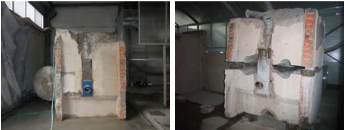
Fig. 20. Segmentation of tank inlets.
