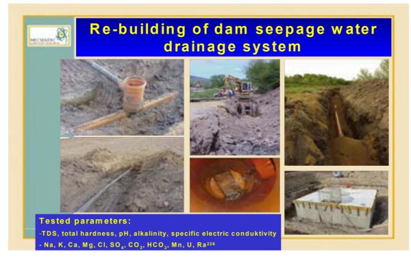
FIG. 2. Re-building of dam seepage water drainage system.
