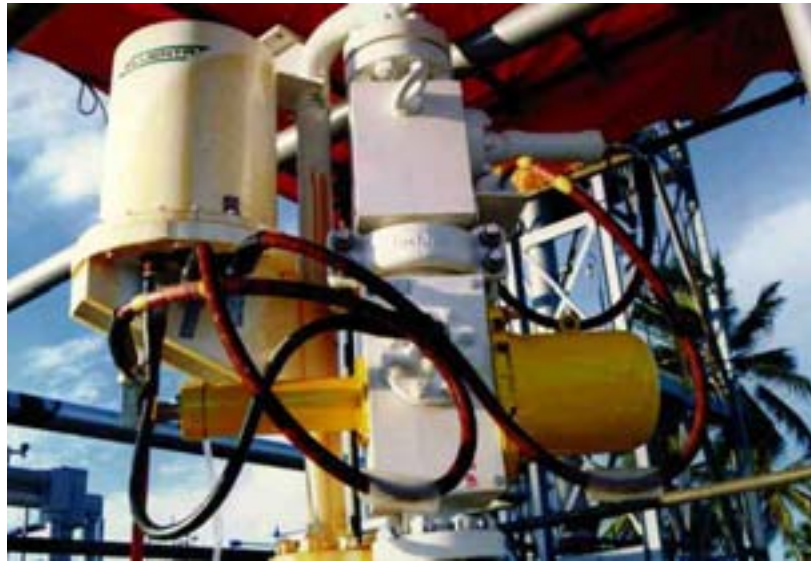
FIG. 13. Multiphase flow meter (MEGRA) installed in oil platform
