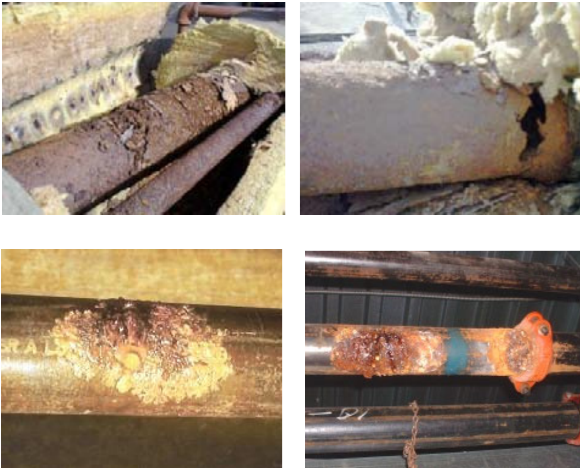
FIG. 1. Corrosion in pipes.
