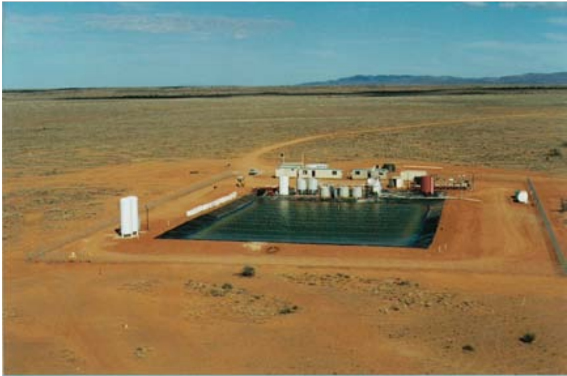
FIG. 7. The Beverley field leach trial plant.
