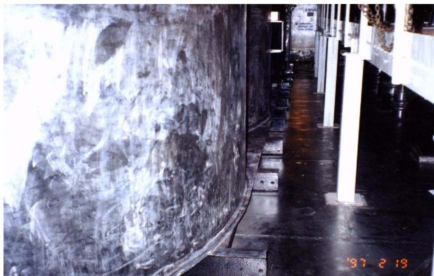
FIG. 4.14. Typical arrangement of the bottom part of multi-cylindrical vertical liquid storage tanks as installed on WWER-440/213 NPPs.
