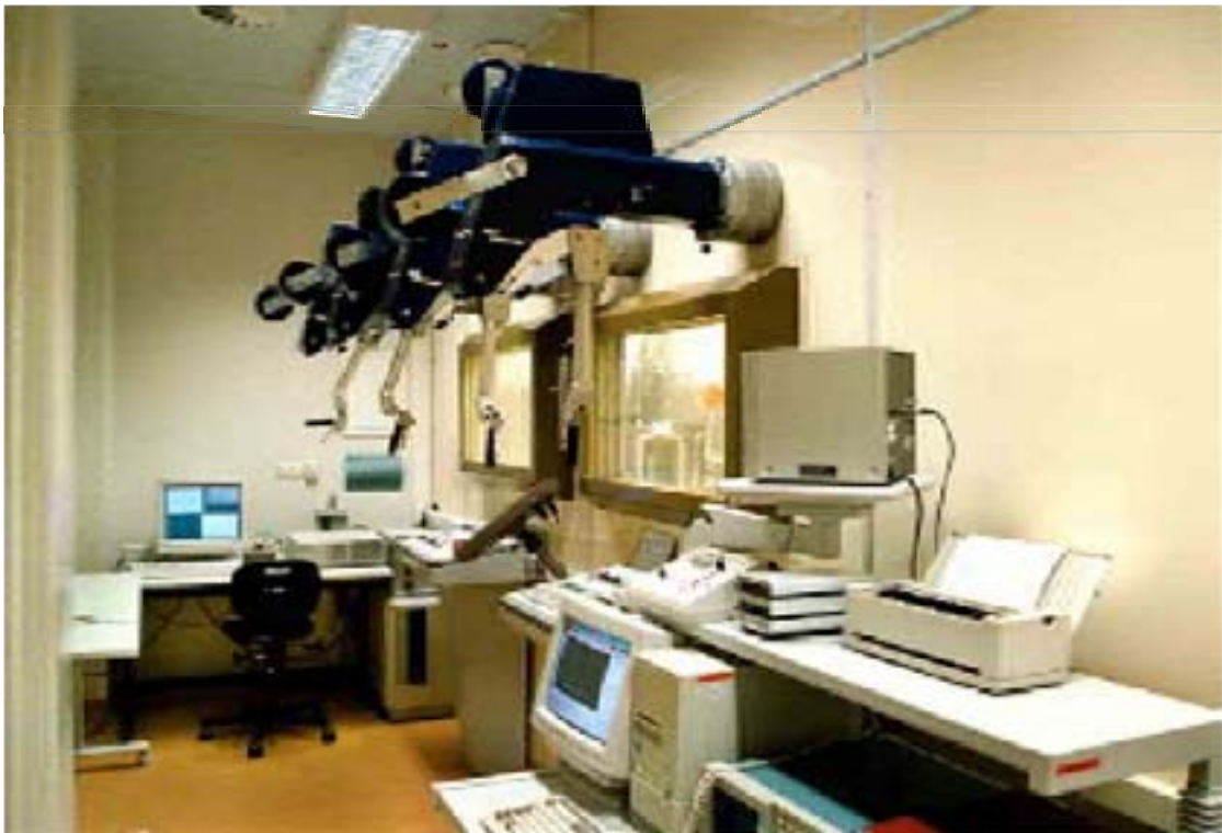
FIG. 11. Hot cell with installed master slave manipulators (Source: Wälischmiller GmbH, Germany).
