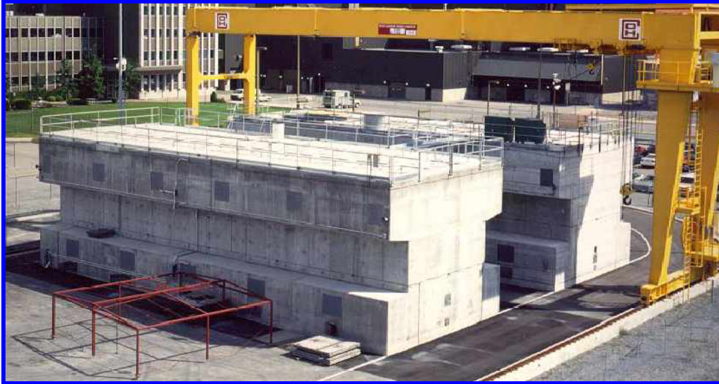
Figure 7-2: MACSTOR dry storage facility (Canada)
