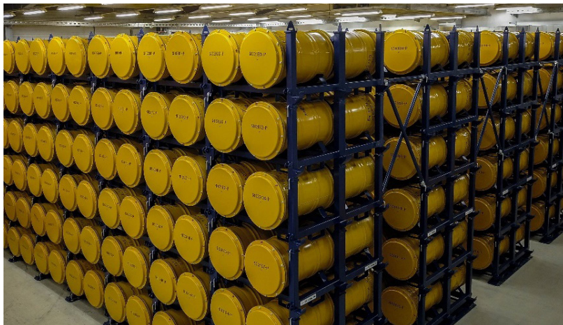
FIG. 30. Conditioned LLW in 200-L drums in an interim storage facility (image courtesy of Nuclear Engineering Seibersdorf).
