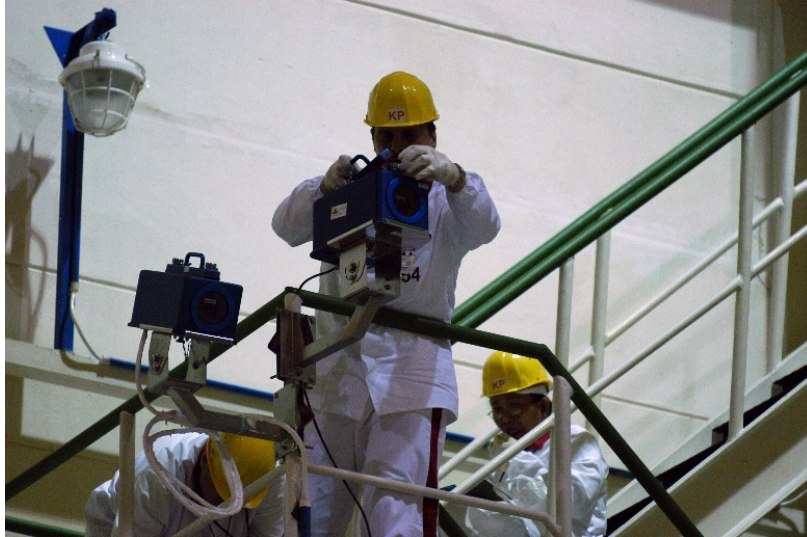
FIG. 10. Installation of a surveillance system.
