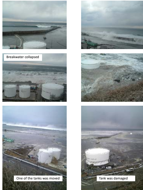
FIG. 21. Situation of damaged structures. Reproduced courtesy of Tokyo Electric Power Company [64].
