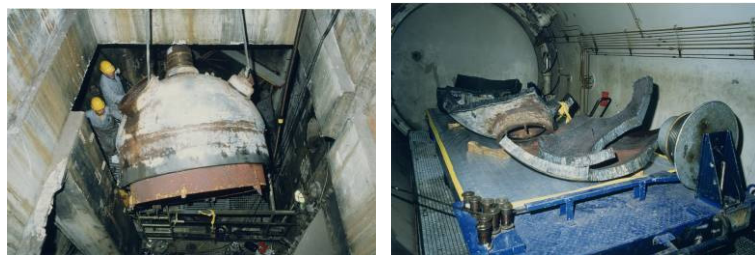
Figure I-6.1 Removal of Steam Converter for further treatment
