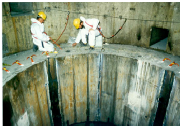
Figure I-8.2 Biological shield removal at HDR using soft explosions.
