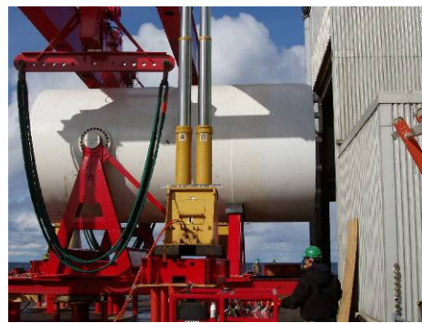
Figure I-1.2 BRP RPV Removal
