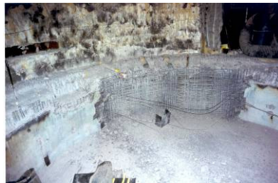
Figure I-8.1 Removal of the KKN biological shield by soft explosions.
