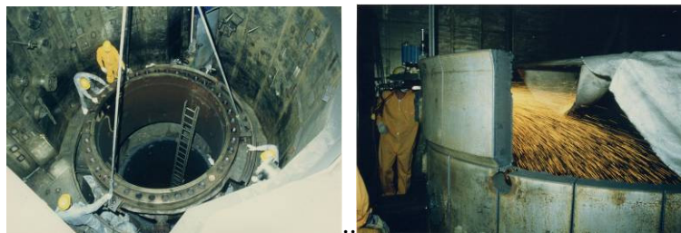
Figures I-6.3 Removal and segmentation of RPV.
