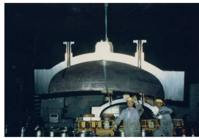
Figure I-6.2 Removal and segmentation of RPV lid.
