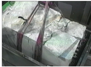
Figures I-8.3 Removal of cut concrete blocks from the WAK reprocessing plant for further treatment at the central waste treatment facility HDB.
