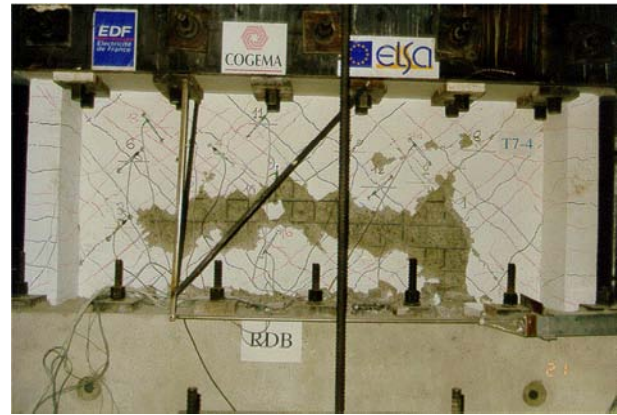
FIG. 14. SAFE crack patterns after testing.
