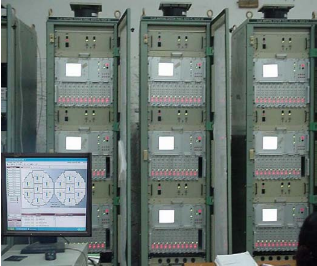
Figure 2: Flux Mapping System for TAPP
