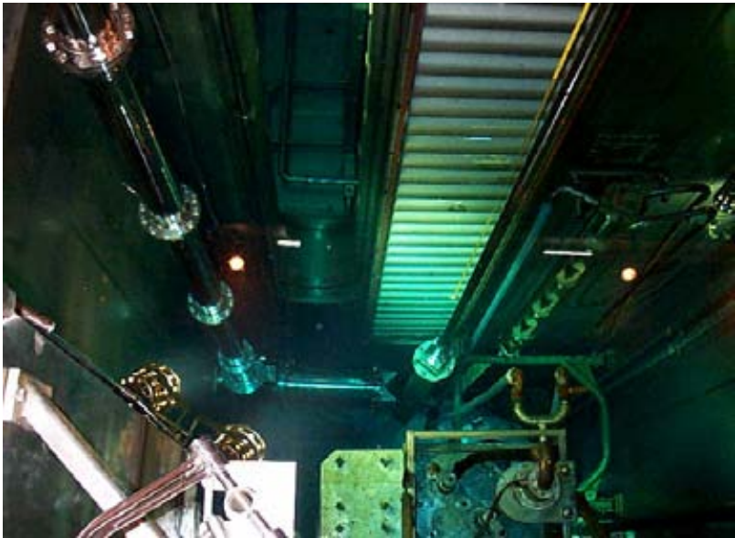
Figure 10. Underwater Gamma Scanning System for Burnup Measurement
