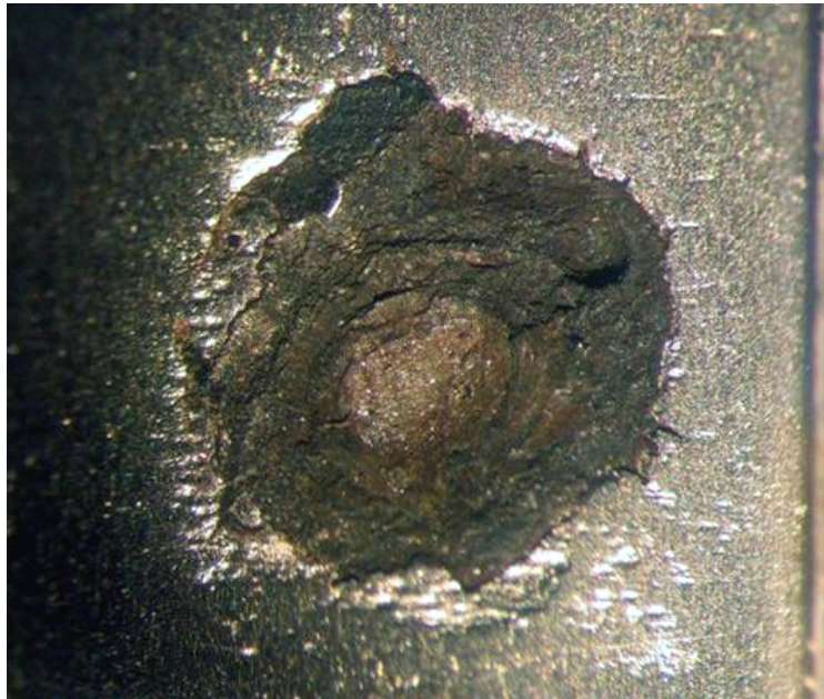
Fig. 7(a). Pitting-surface appearance.
