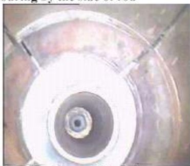
G. Clean Freeze Valve after normal pouring
