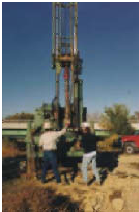
Fig. XIII-10. A drill rig is positioned prior to drilling a monitor well at a remediation site.
