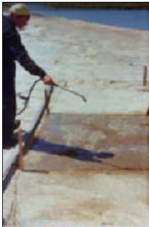
Fig. VII-54. The process of application of polymer coatings.
