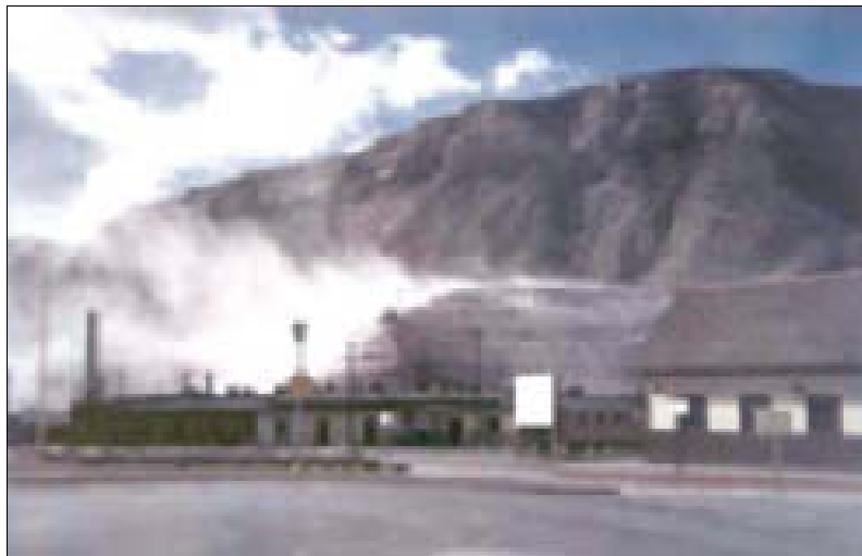
Fig. XIII-8. Windblown tailings increase both the areal extent of contamination and the area that requires characterization.
