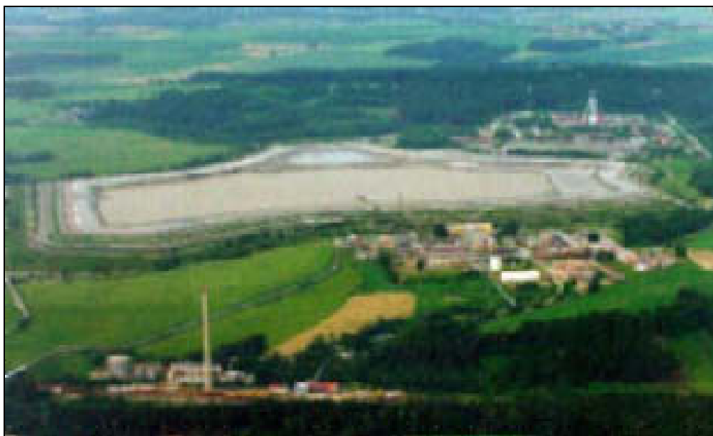
Fig. IV-27. View of the tailings pond K1 Rožná – aerial photograph.
