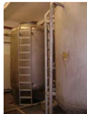
FIG. 3. A view of decay tanks installed in a medical establishment.
