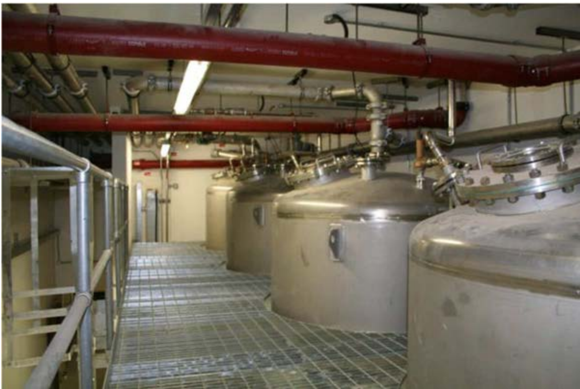
FIG. 16. The upper part of the decay tanks viewed from the inspection gantry.
