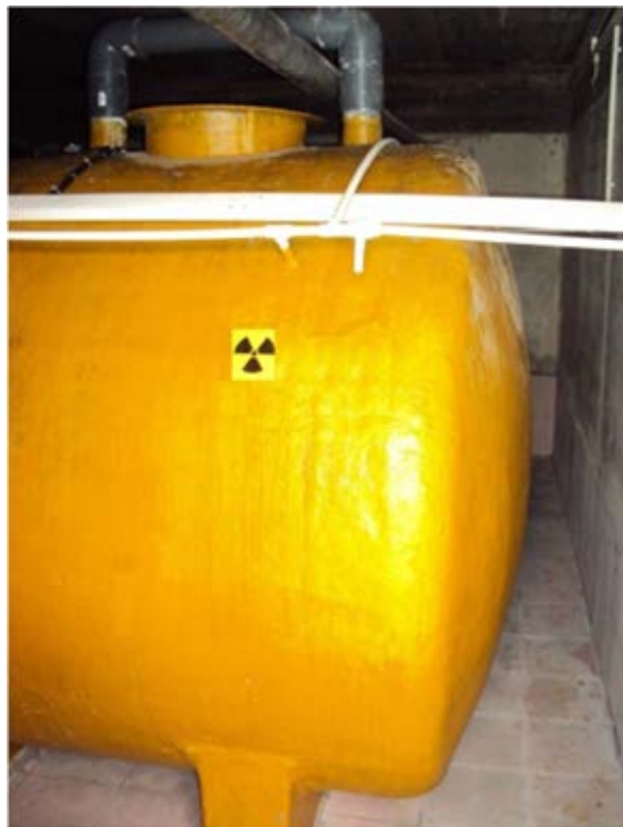
FIG. 20. View of tank systems installed in a medical establishment.
