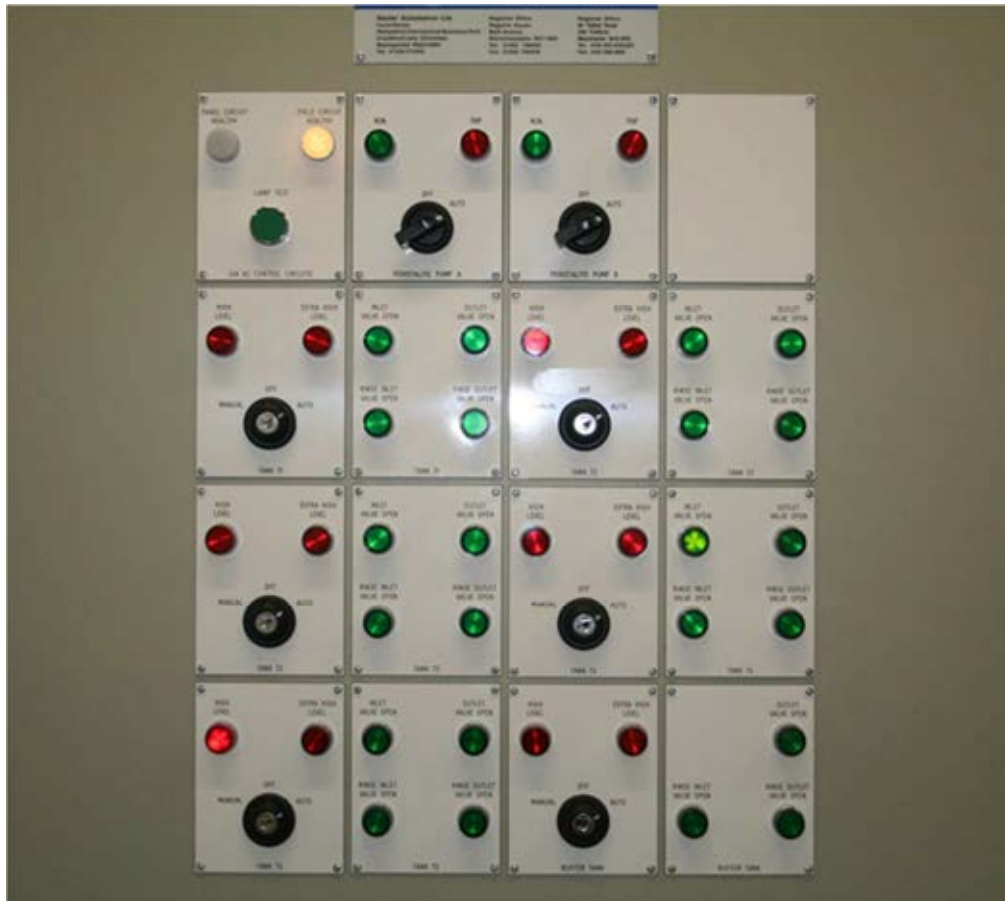
FIG. 10. The control panel with key access manual override option.
