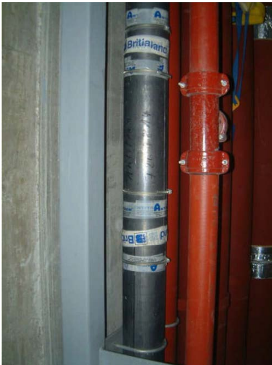
FIG. 12. The pipe on the right is the main riser and the lead clad pipe on the left is carrying active waste to the tanks from the radiotherapy patient bathroom.
