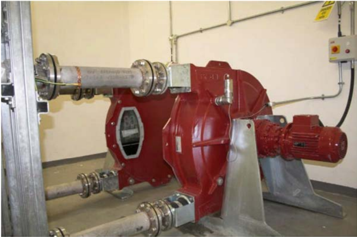
FIG. 14. The two peristaltic pumps used to pump the liquid from the tank.
