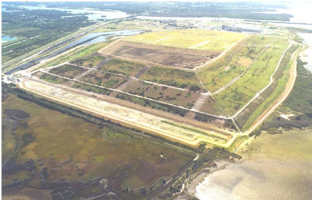
FIG. 11. Phosphogypsum stack being converted into a permanent disposal facility (courtesy: Fertiberia, Spain).
