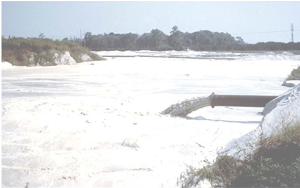
FIG. 10. Phosphogypsum tailings being returned to the mining void (courtesy: Florida Industrial and Phosphate Research Institute, USA).
