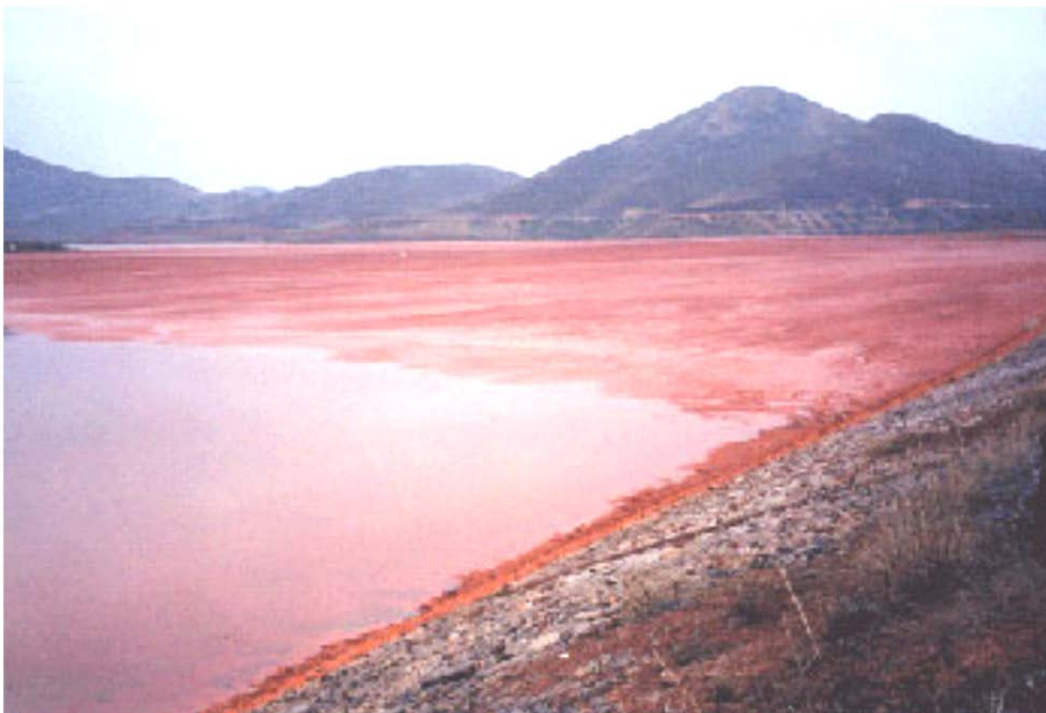
FIG. 8. Disposal of bauxite tailings in an engineered containment.
