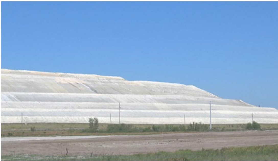
FIG. 2. Stockpiling phosphogypsum in a stack (courtesy: Florida Industrial and Phosphate Research Institute, USA).
