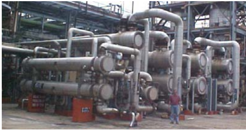
FIG. 43. Bank of heat exchangers in refinery where radiotracer test was carried out to search for leaks
