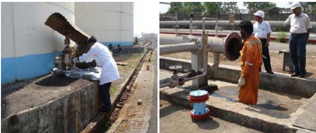
FIG. 73. Radiotracer introduction (left) and pig launcher (right)
