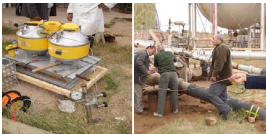
FIG. 63. Injection of the radiotracer gas methylbromide from the generator to the pipeline using a manual air pump with manometer
