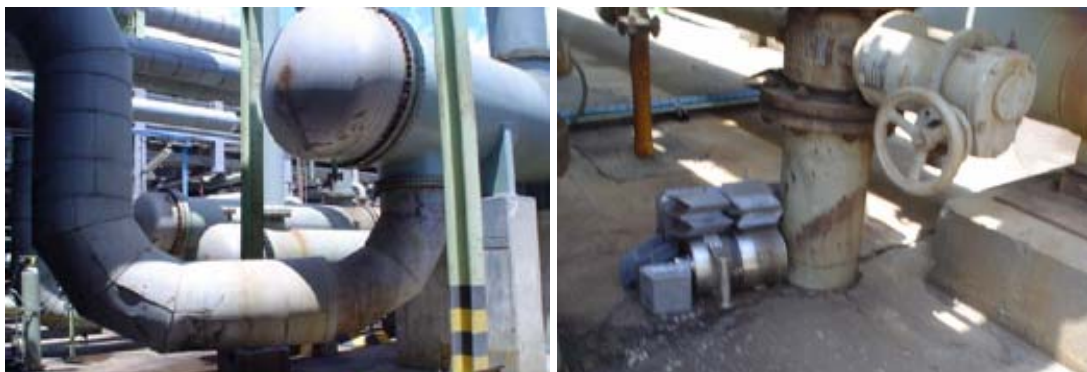
FIG. 33. The shell and tube type heat type exchanger and shielded detector
