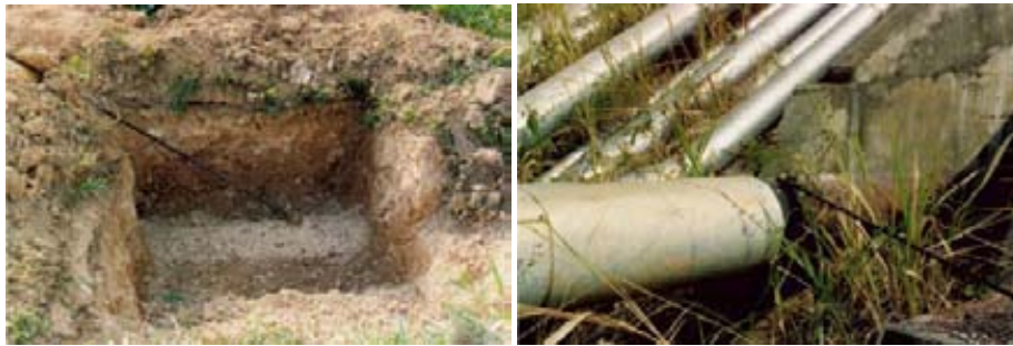
FIG. 58. ^{60}\text{Co} markers installed in a pit (left) and on the pipeline(right)
