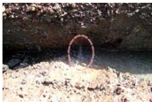
FIG. 75. Leak visually confirmed
