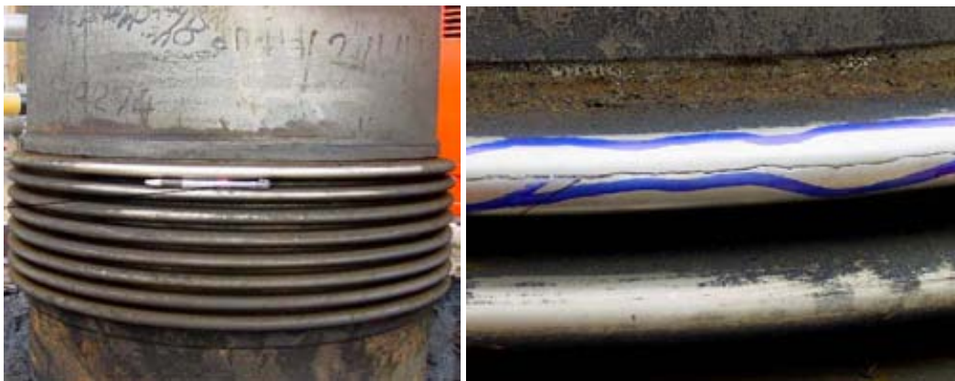
FIG. 29. Visual inspection after shut-down shows leak point
