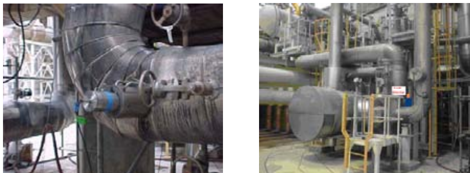
FIG. 16. NaI probes with lead collimator mounted at the outlet of a heat exchangers
