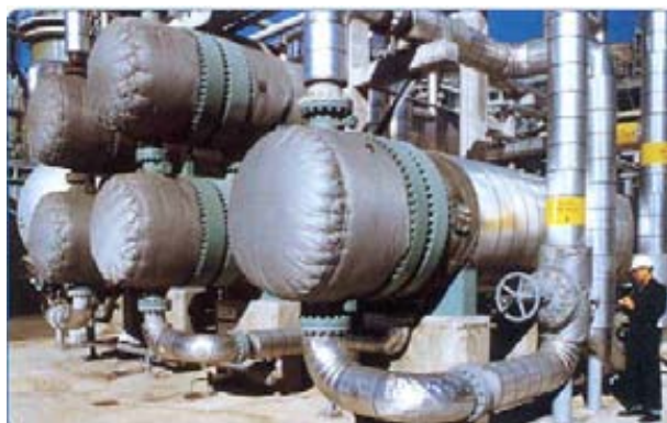
FIG. 50. Bank of heat exchangers
