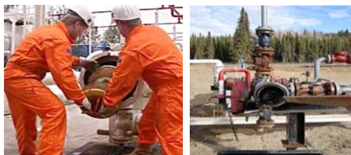
FIG. 57. Inserting the pig into a pig launcher of a pipeline
