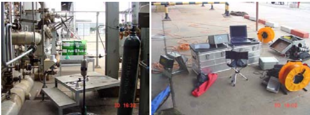
FIG. 26. Injection facility(left) and data acquisition system (right)
