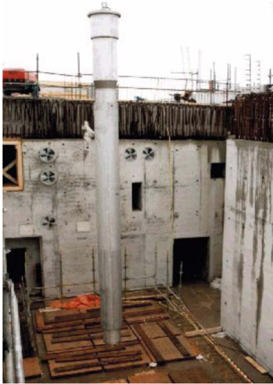
FIG. 10. Fitting of a storage pit during the construction of the HABOG facility [10].
