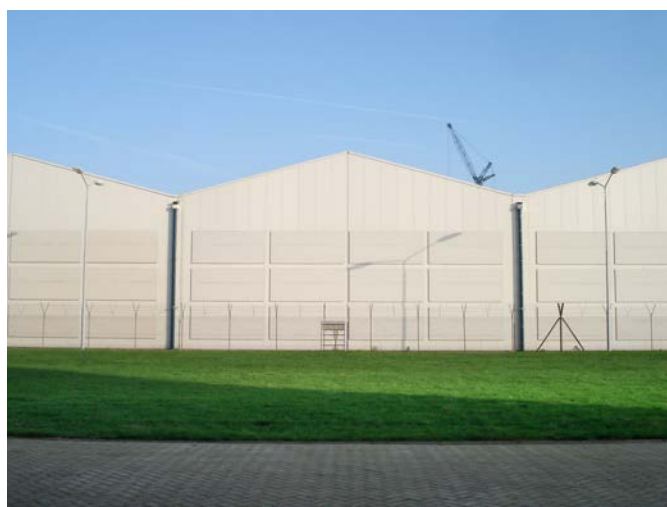
FIG. 4. Storage facility for NORM waste.
