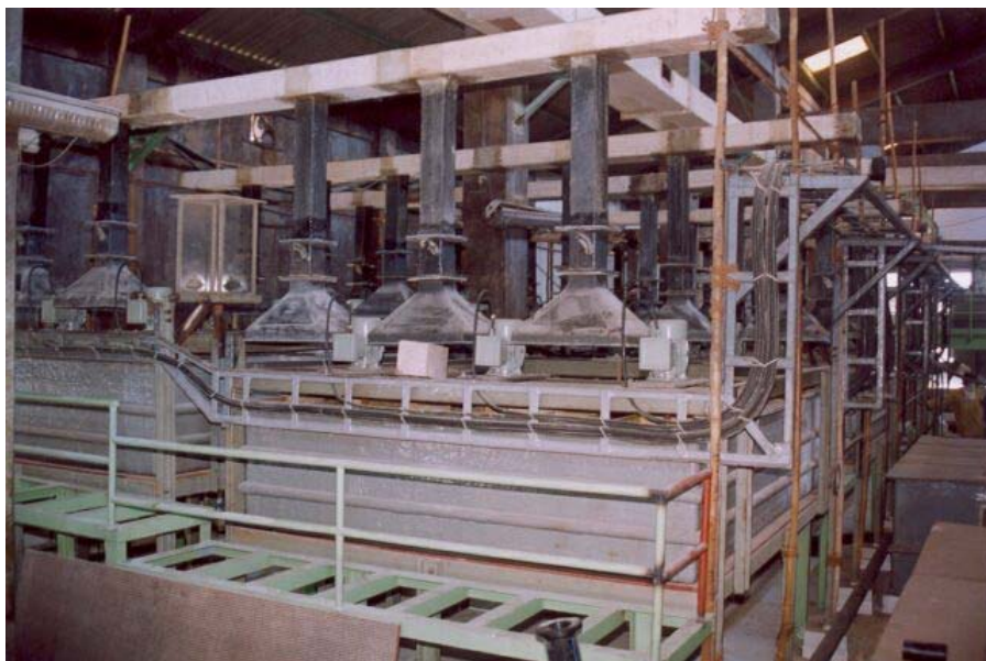
FIG. 20. Mixer settlers used for the separation of rare earths via solvent extraction.
