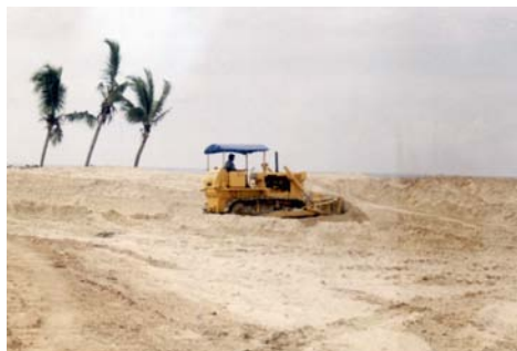
FIG. 15. Backfilled mined out area.
