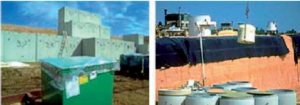
FIG. 12. View of the two types of modular concrete canister facilities for LLW disposal at the Barnwell site, South Carolina.
