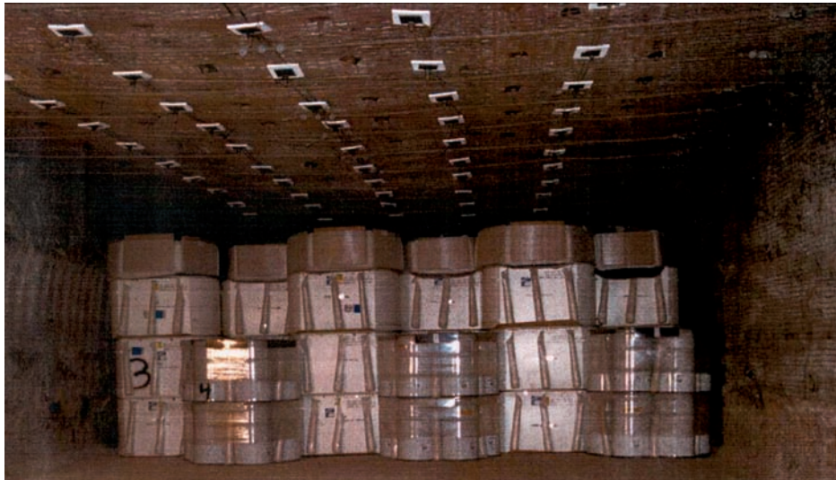
FIG. 10. Photo of CH-TRUW and magnesium oxide backfill emplaced in one of the disposal rooms of the WIPP repository (courtesy of USDOE).
