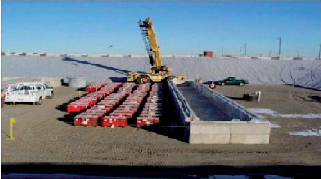
FIG. 11. The shallow land burial facility for LLW at the 200 West Area at the Hanford site.
