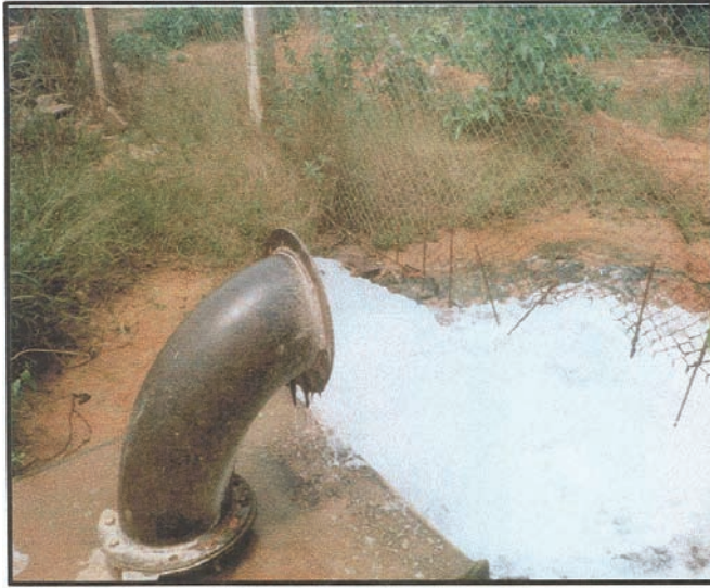
FIG. 1. An Oji artesian borehole discharging freely.
