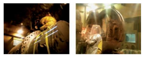
FIG. 4. Installation of the diamond rope saw in the working caisson and thermal cutting of the low activated part of the KNK reactor rotary lid.
