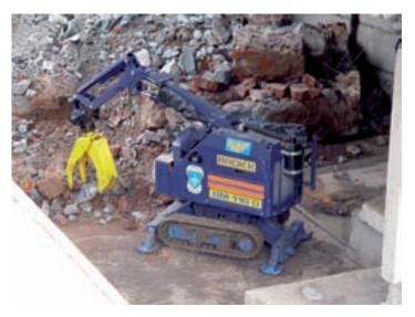
FIG. 2. Removal of waste using robots.
