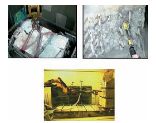
FIG. 5. Treatment of the alpha contaminated blocks of WAK with a remote controlled excavator equipped with an adaptor for a pneumatic hammer.
