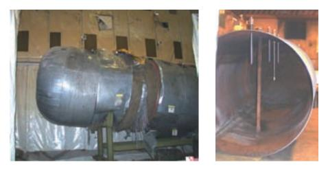
FIG. 2. Sodium discharge tank during spray moistening for sodium conversion with continuous monitoring of the hydrogen concentration.
