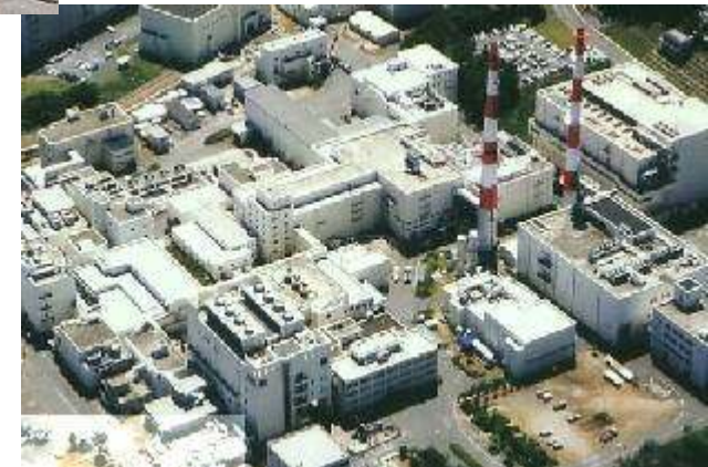
Tokai Reprocessing Plant (JAEA)
