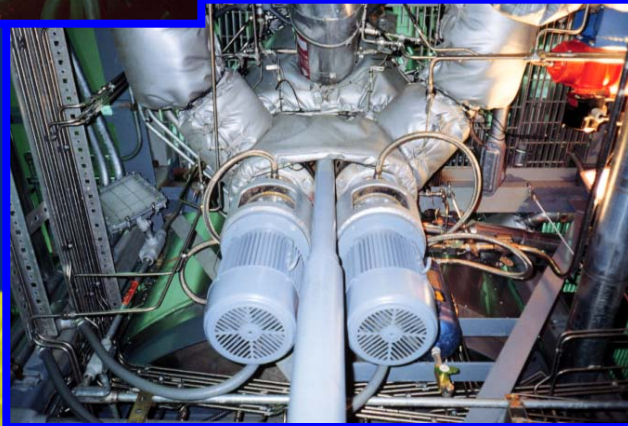
Reactor Coolant Pumps
