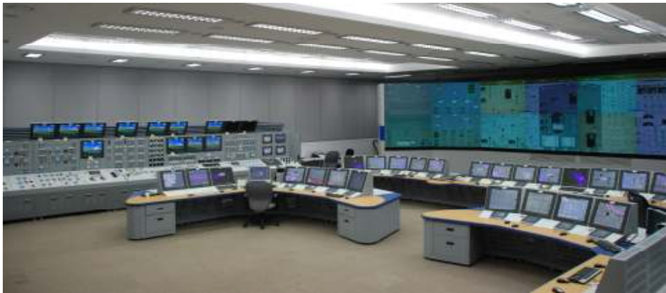
Fig.1 Main control room overview of performance test facility
