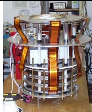
Figure 2: Interior details of 3:1 step-down transformer driver
