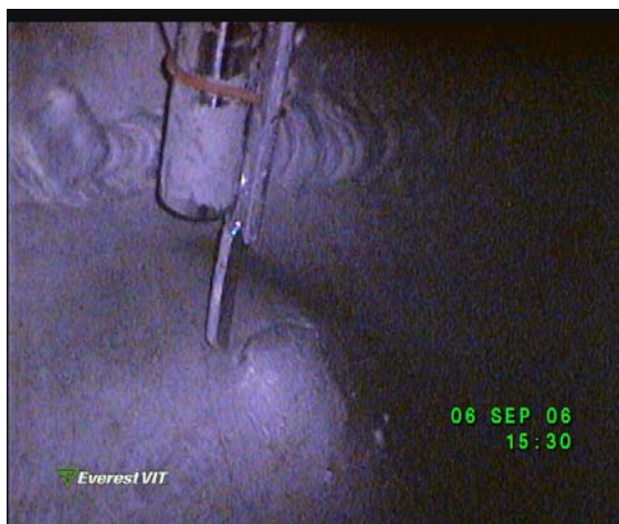
Fig. 3. Ultrasonic thickness measurement of tank wall.
